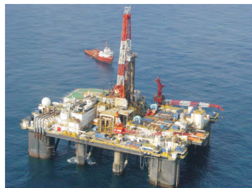
流花4-1电飞缆抢修/流花11-1深水动态缆 LH4-1 Flying Leads Repair/LH11-1 Dynamic Cable
