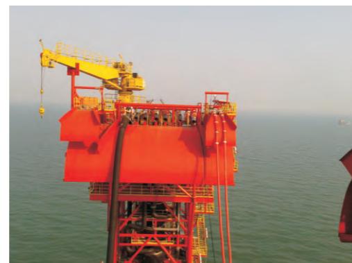
渤中25-1软管脐带缆 BZ 25-1 Hose Umbilical
