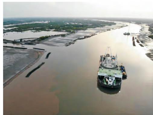
越南BINH DAI海上风电项目/35kV Vietnam BINH DAI Offshore Wind Power Project
