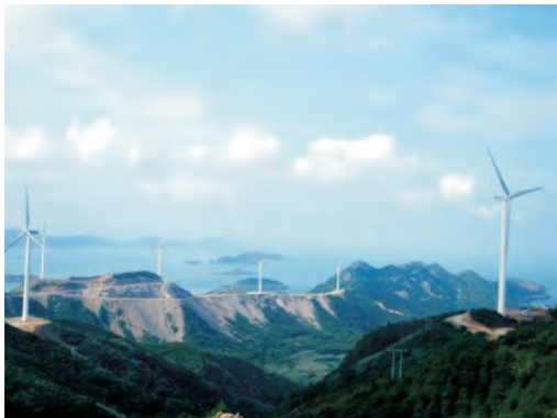
霞浦浮鹰岛风电场项目/110kV Xiapu Floating Eagle Island Wind Farm Project
