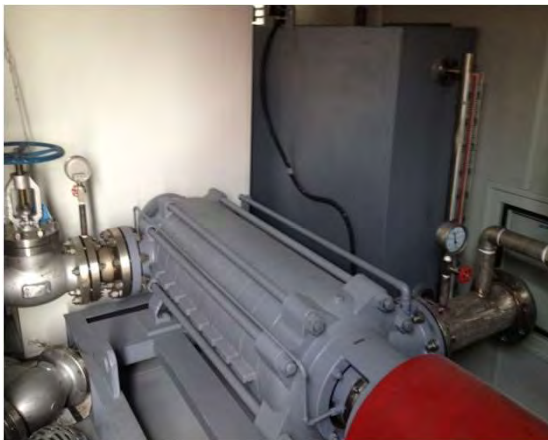
Pigging Pump Rated Capacity: 150m 3 /h&250m 3 /h Head of Delivery: 400m
