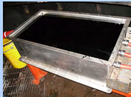
Sealed vertical and horizontal junction boxes
