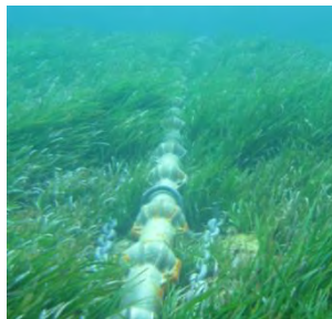
Safety on seabed
