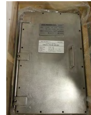
ATEX Certified Junction boxes for power and fibre optic
